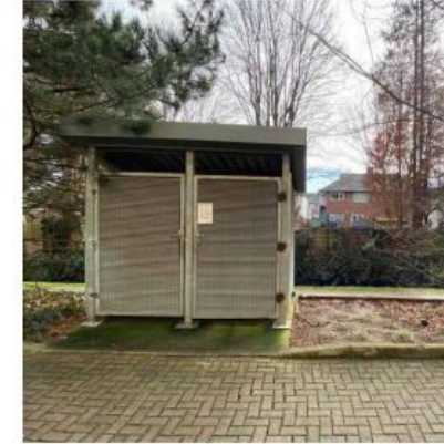
Existing Bin Stores - Capacity for 2no. 1100L bins
